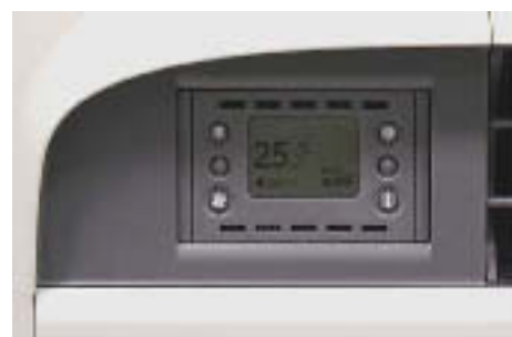
DISPLAY CONSOLE INSTALLED ON A SPHERA FAN COIL UNIT
