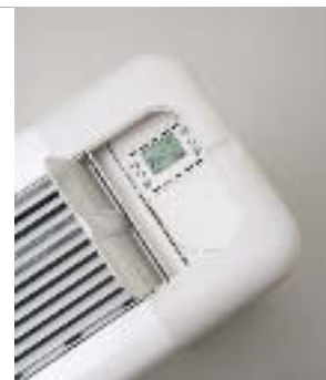
DISPLAY CONSOLE INSTALLED ON A FAN COIL UNIT
